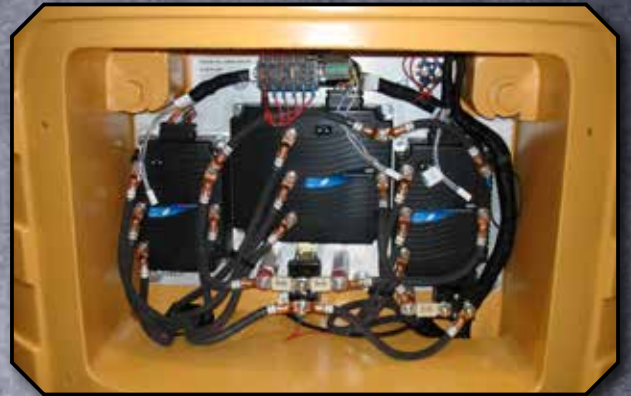
Rear Controller Compartment and Counterweight
